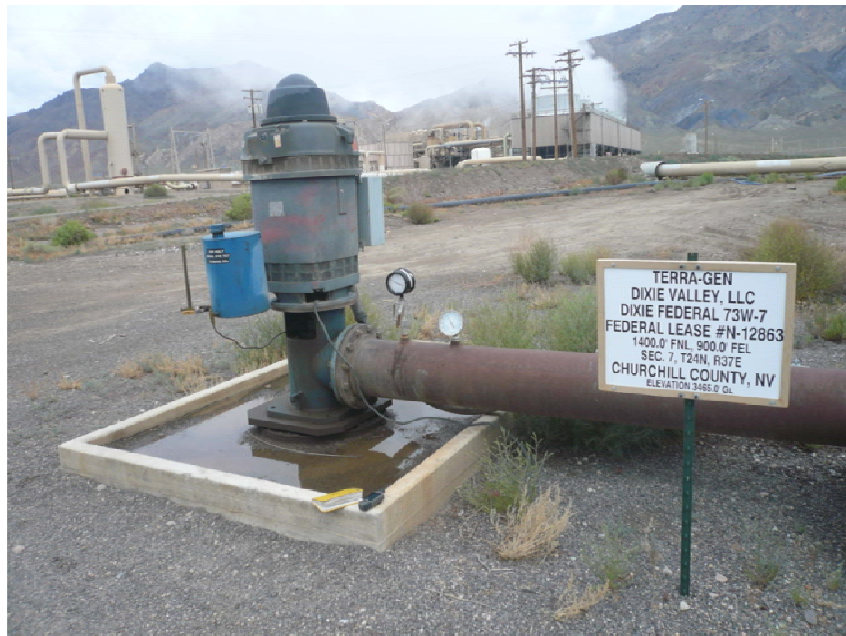
Figure 3: Digital image of Well 73W-7 with the Dixie Valley Power Plant in the background.
