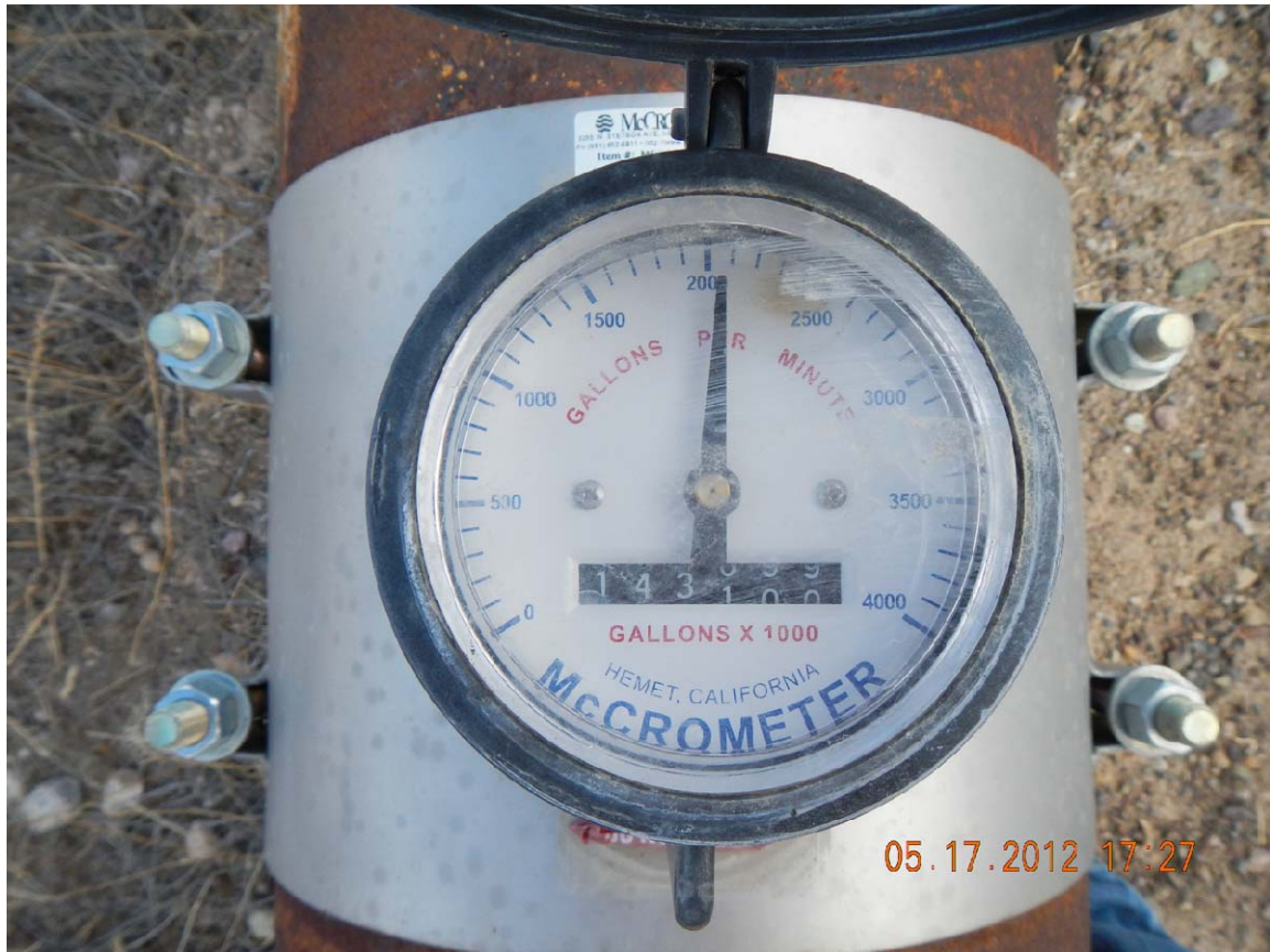
Figure 11: Image of flow meter on Ag. Well #2, Lincoln Ranch.
